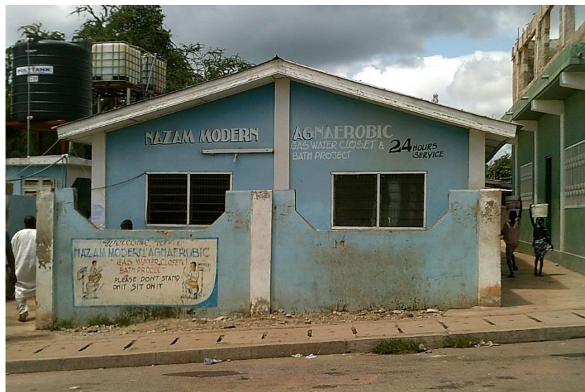
Figure 15: Bio-Digester Public Sanitation Block in Obuasi, Ashtanti, Ghana. Constructed by Impact Environmental Ltd.
