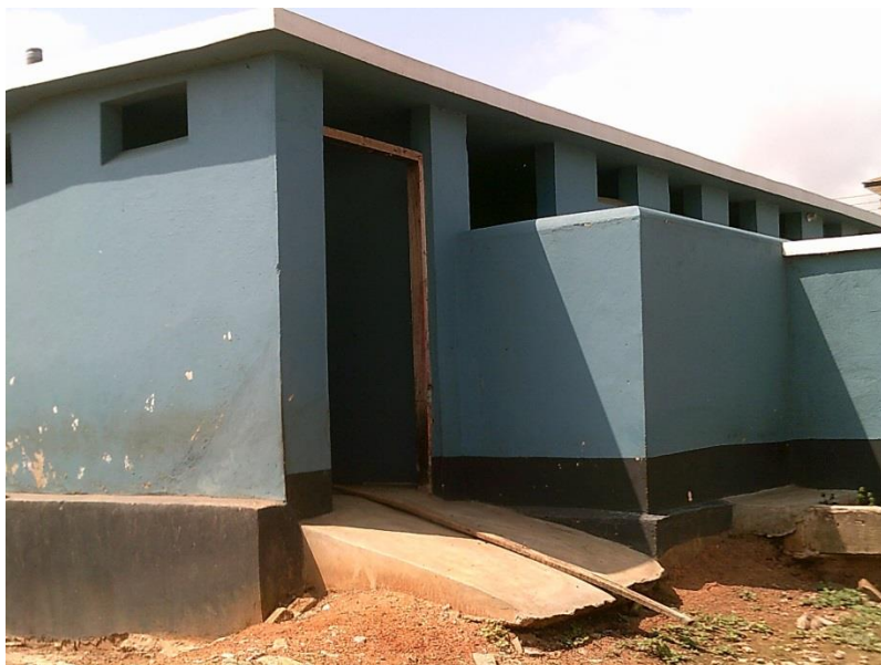
Figure 11: Sanitation Block in Ayigya Neighborhood
